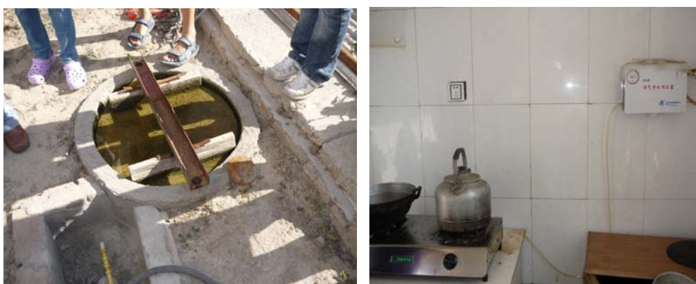
Figure 4: Marsh gas tank and use of methane in Shandong province
