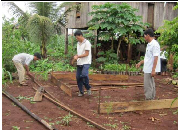
Photo 7 Housing location preparation
